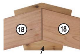
Adjust the trusses until centered left / right and up / down on the pentagon cap. Place one bottom board (Item 6) under each truss. This will help level the trusses.
